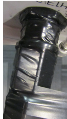
Figure 30: Wrapping the Connector with Electrical Tape
