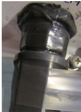
Figure 28: Wrapping the Connector with Rubber-splicing or Self-amalgamating Tape
